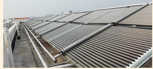
In Nanjing, China, a solar water heater on the roof of the recently completed factory provides hot water for the whole dormitory, reducing energy consumption
