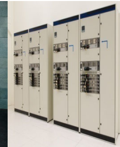
Building Automation & Security
