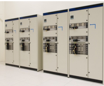
Building Automation & Security
